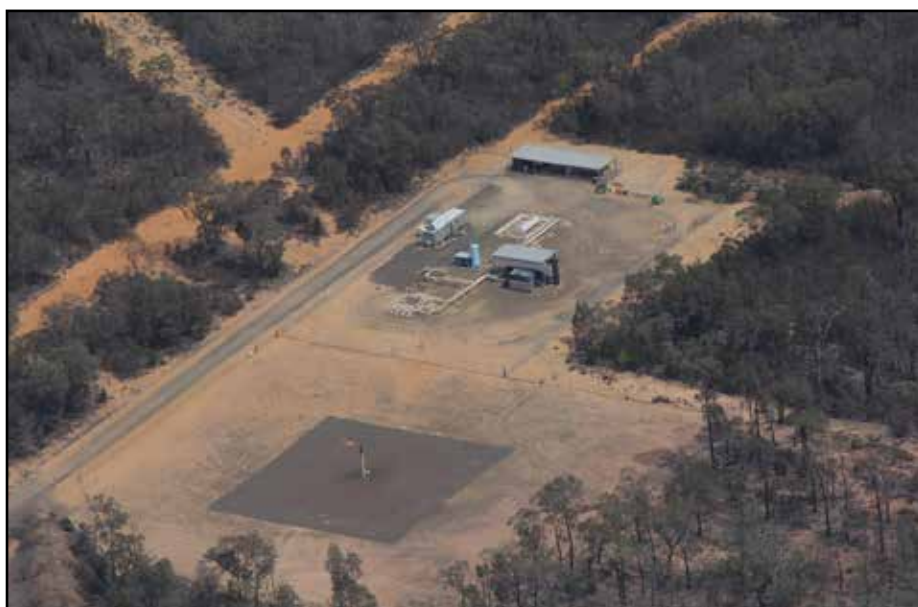
A flare and compressor station in the Pilliga. Photo: North West Protection Advocacy
