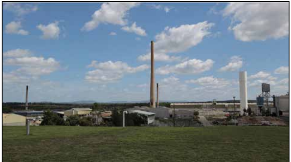
Kurri Kurri aluminium smelter – the chimney stacks have now been demolished.
