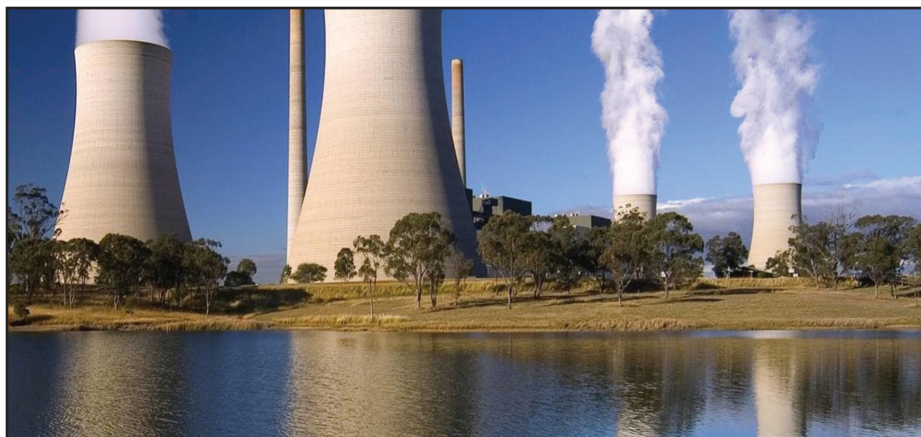
Liddell Power Station shares cooling towers with neighbouring Bayswater, making it difficult to separate the generator and sell it. Photo: AGL Macquarie
