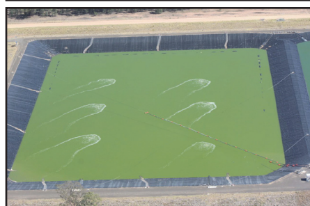
The irrigation area, on April 14, 2018, and (below) an empty brine pond. Photos: Wando Conservation and Cultural Centre
