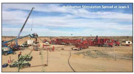
Halliburton contractors fracking Strike's Jaws-1 CSG well using an extreme new technique. Photo: Strike Energy
