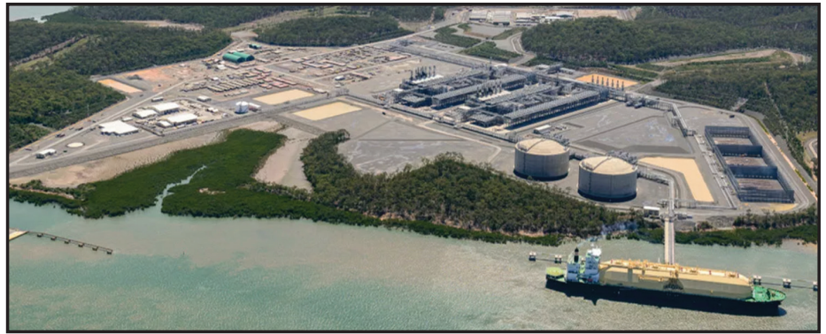
Australia Pacific LNG's Curtis Island plant, Gladstone. Photo: APLNG
