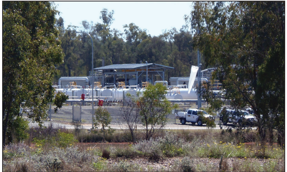
APLNG's Talinga gas plant, Darling Downs, QLD, includes a compressor station.
