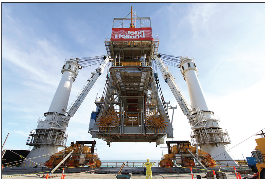
Construction company John Holland in action during the upgrade of Adani's Abbot Point coal port. The two companies ended up in court over the work, with Adani winning costs. Photo: John Holland
