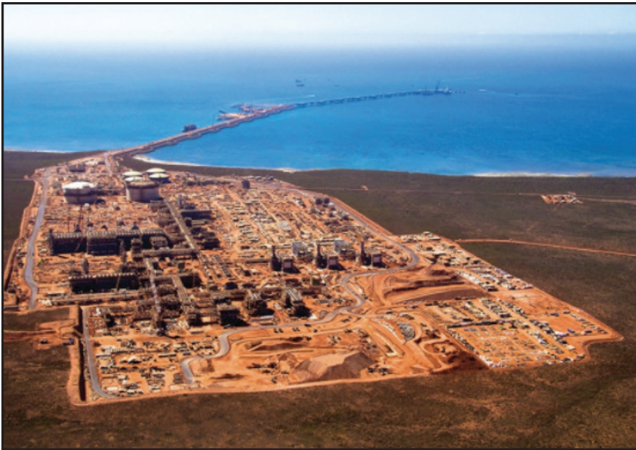
Exxon Mobil Australia's WA Gorgon project. Photo: Exxon Mobil
