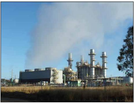
QGC's 140 MW Condamine Power Station, 8km east of Miles, is powered by CSG running two gas turbines and one steam turbine. Photo: Contributed
