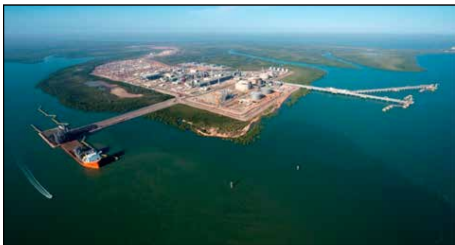
INPEX's Bladin Point onshore gas facility in Darwin Harbour. Photo: INPEX
