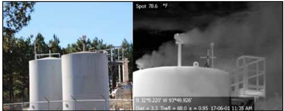
Left: gas storage tanks as they look to the naked eye. Right: An infrared camera shows methane gas being vented from the tank. Photos: Robert Howarth, Biogeosciences
