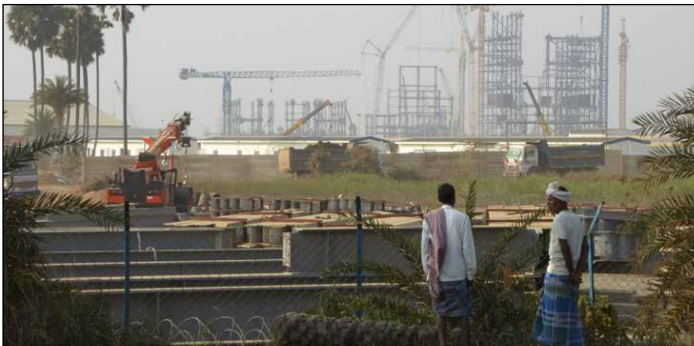
Indian traditional farmers looking at Adani's Godda power plant, being built to burn Australian coal. Photo: Geoff Law
